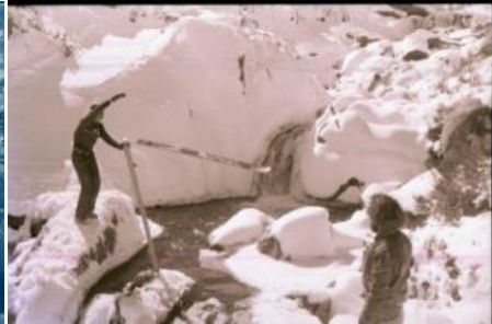
Merritt's Creek Cross
