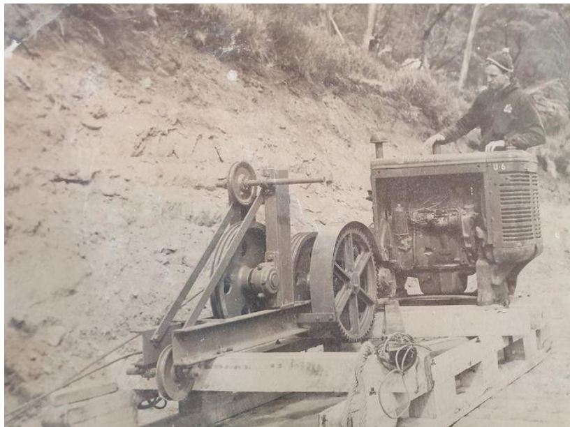
The first Ski Lift and International Harvester Tractor engine and gearbox and locally produced Drive unit - Danny Collman on the back as it is self-winched up to position - 1957
