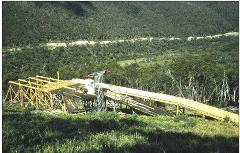
Ramshead Top Station Platform which was later moved moved to a higher position due to the build up of snow
