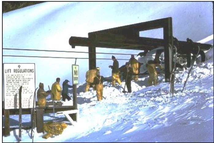
Volunteers digging out Ramshead Top Station (1964)
