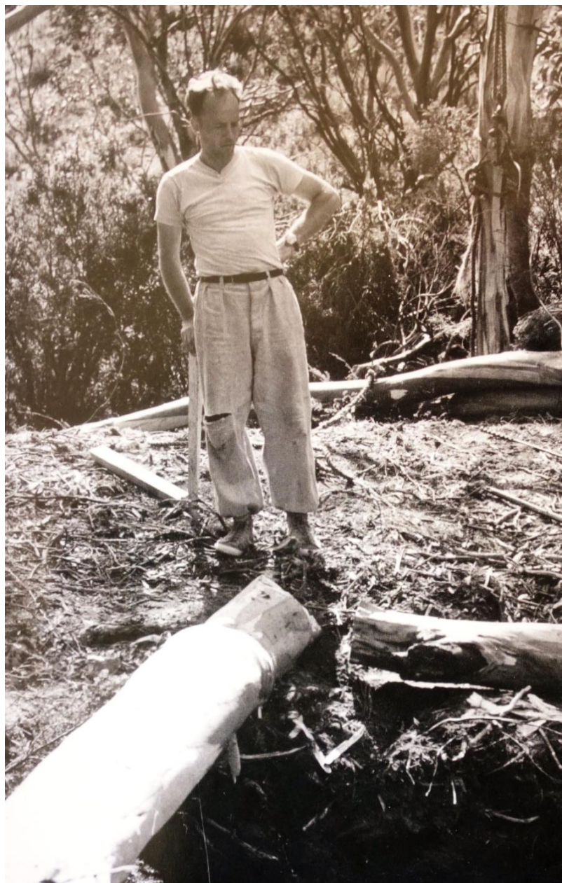
Tony Sponar building a bridge over the Thredbo River - 1956
